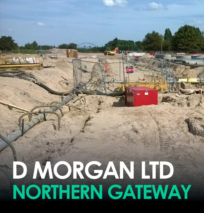
Temporary wellpoint dewatering to enable construction of a foul drainage system
