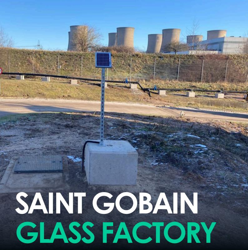
Permanent dewatering solution to the rising groundwater issues at a glass manufacturing facility within a Groundwater Protection Zone
